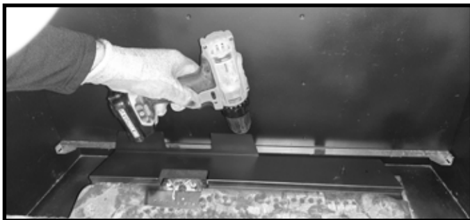
Figure 3 Install Back Refractory Support
