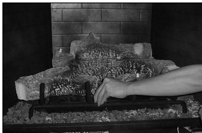
Figure 12.3 Placement de la vermiculite
