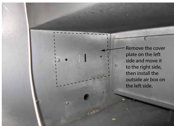
Figure 3.14 Remove Cover Plate (Left Side)
