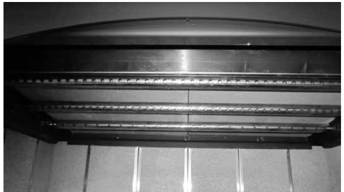
Figure 4.8 Reinstall Baffle Boards
