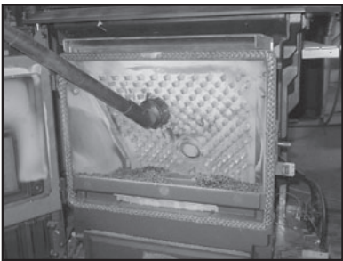
Figure 28.1 - Example of a dirty heat exchanger
