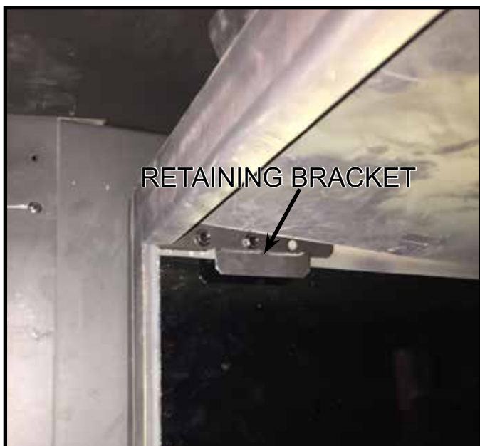
Figure 11.8 Retaining Bracket Installation - Side Panel
