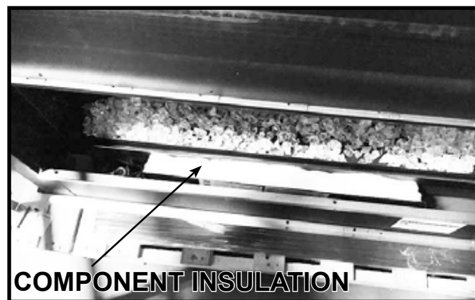
Figure 11.3 Component Insulation Location
