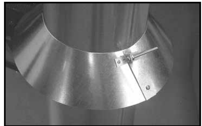
Figure 7.14 insert Bolt into Brackets
