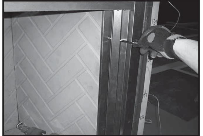
Figure 9. Loosen Refractory Retaining Strip
