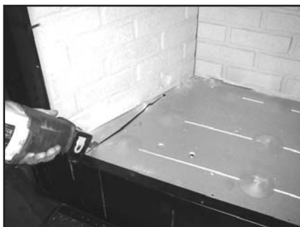
Figure 11.2. Using a saws-all, cut out the floor.
