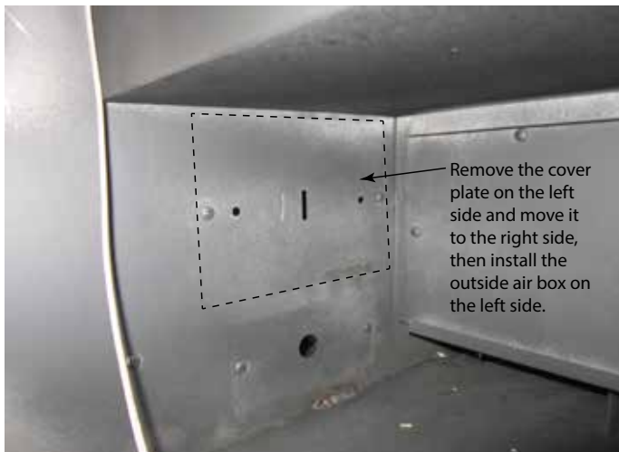
Figure 3.14 Remove Cover Plate (Left Side)
