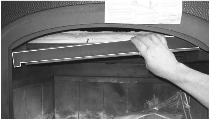
Figure 4.8 Removing Baffle Protection Channel
