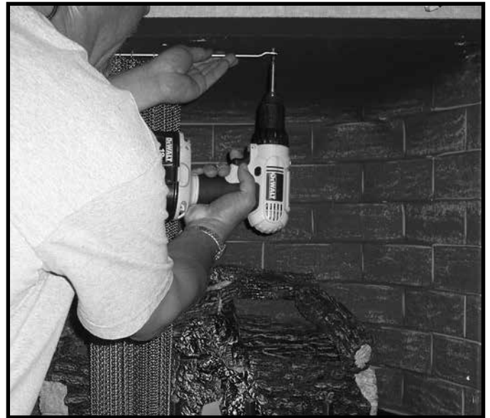
Figure 8.17 Fasten Screen Rod to Firebox Top
