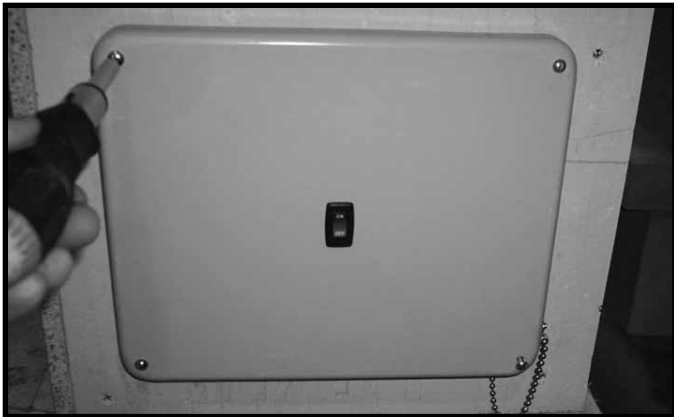
Figure 5.1 Remove Control Cover
