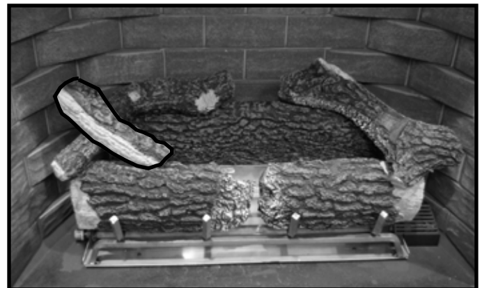
Figure 8.10 Place Top Log on Left Side
