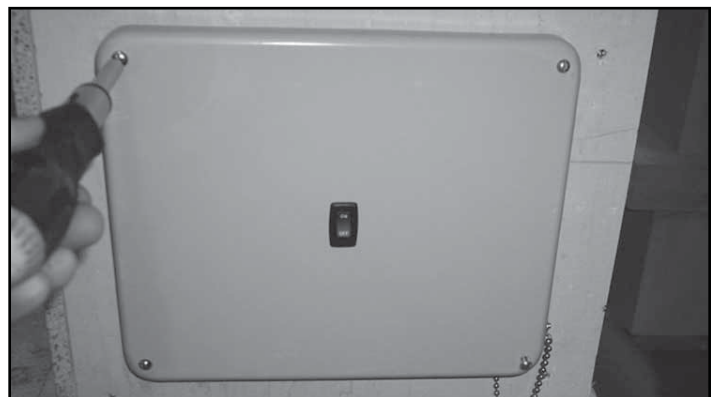
Figure 9. Replace Control Cover
