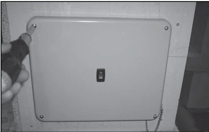
Figure 1. Remove Control Cover
