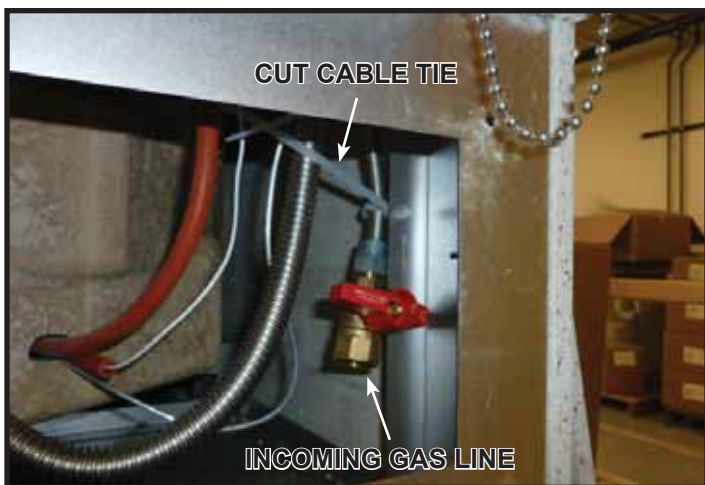
Figure 5.2 Connect Incoming Gas Line to Manual Shutoff Valve
