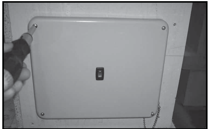
Figure 6.11 Replace Control Cover
