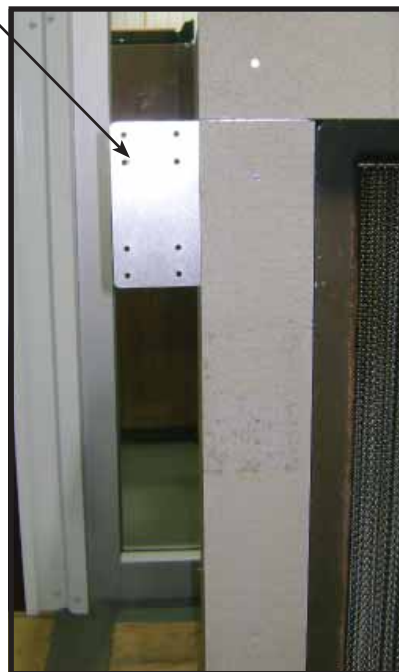
Figure 4.1 Positioning and Securing Nailing Tab
