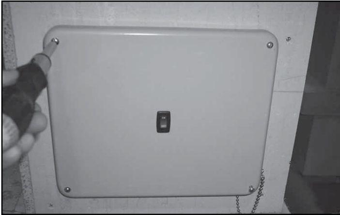
Figure 6.3 Remove Control Cover
