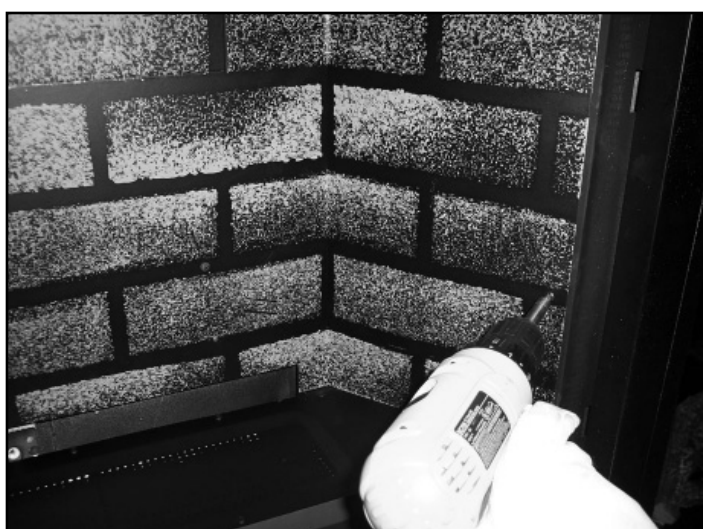
Figure 2.8 Install Screws
