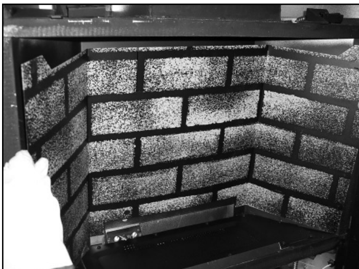
Figure 2.5 Install Refractory in Appliance
