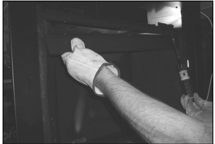
Figure 1.9 Remove Glass Heat Shield
