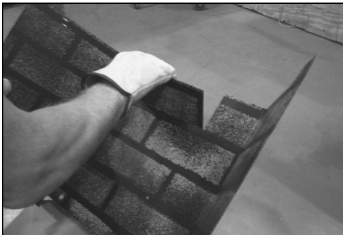
Figure 2.4 REAR VENT ONLY - Fold Flue Visor Cover
