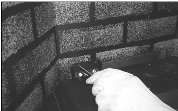
Figure 3.1 Replace Pilot Shield
