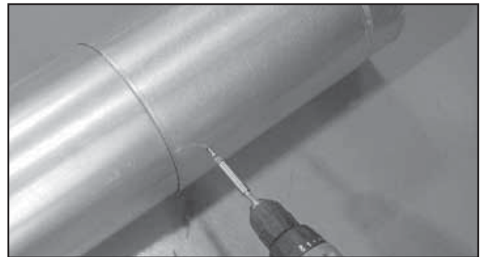
Figure 10.7 Screws into Slip Section
