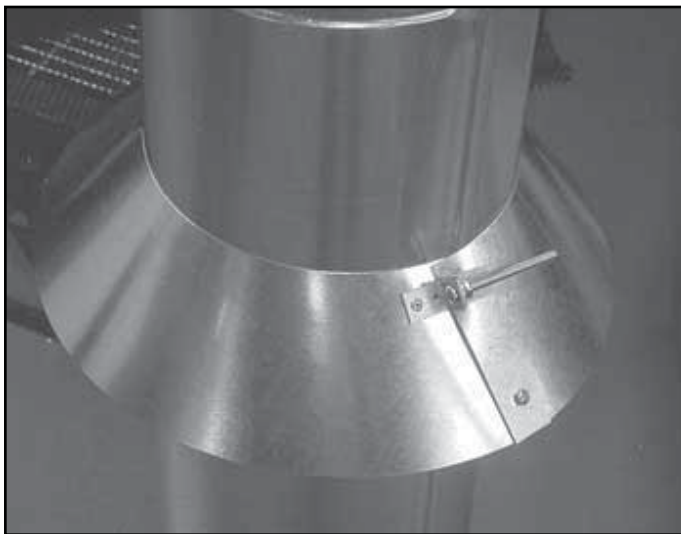
Figure 10.17 Assembling the Storm Collar Around the Pipe
