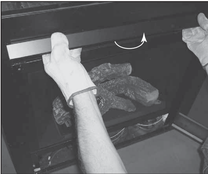
Figure 15.9 Installing Hood
