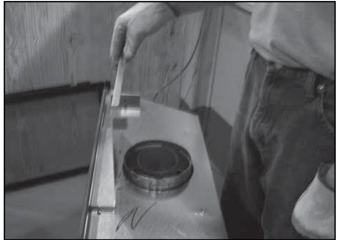
Figure 9.4 Bend Heat Shield
