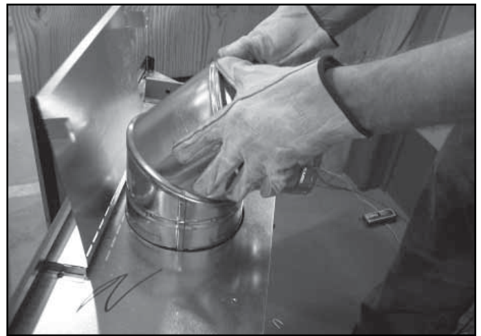
Figure 9.5 Begin Vent Installation
