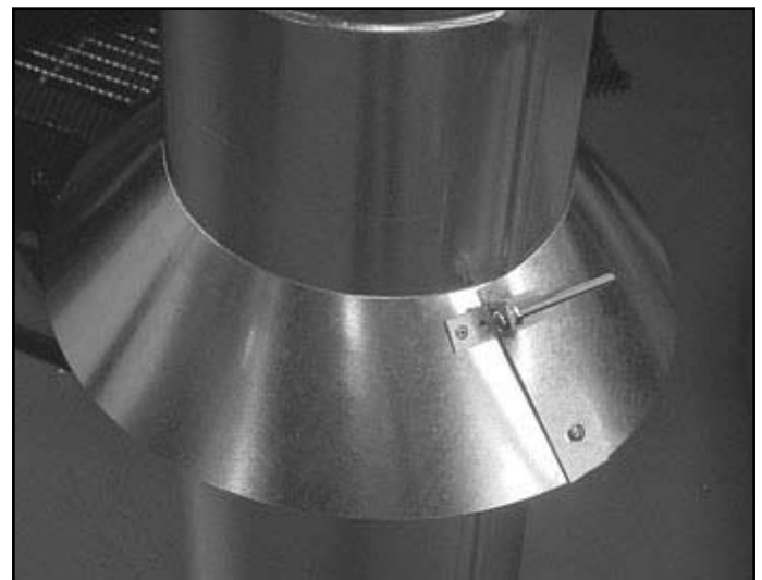
Figure 10.12 Assembling the Storm Collar Around the Pipe
