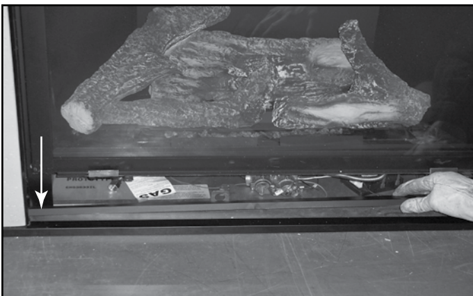
Figure 15.7 Place Floor Cover
