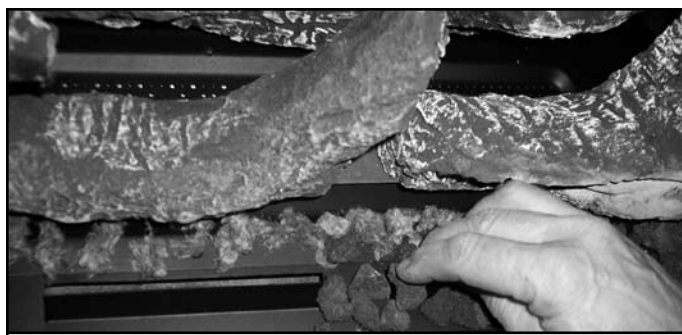
Figure 15.5 Placement of Lava Rock
