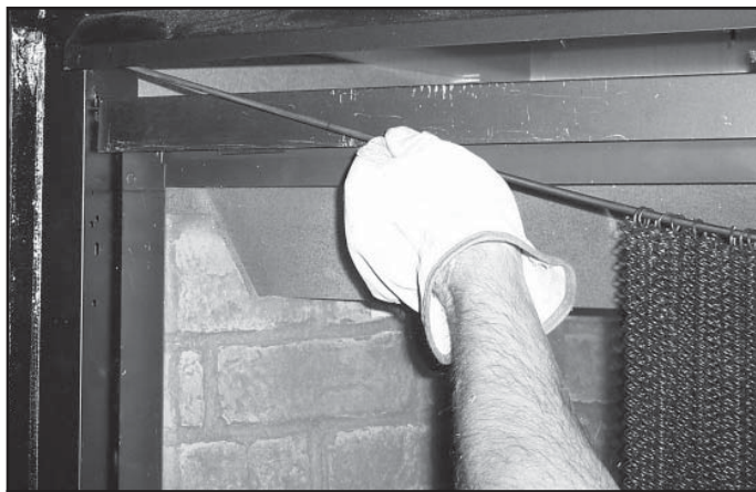
Figure 14.12 Insert Rod Into Side Columns
