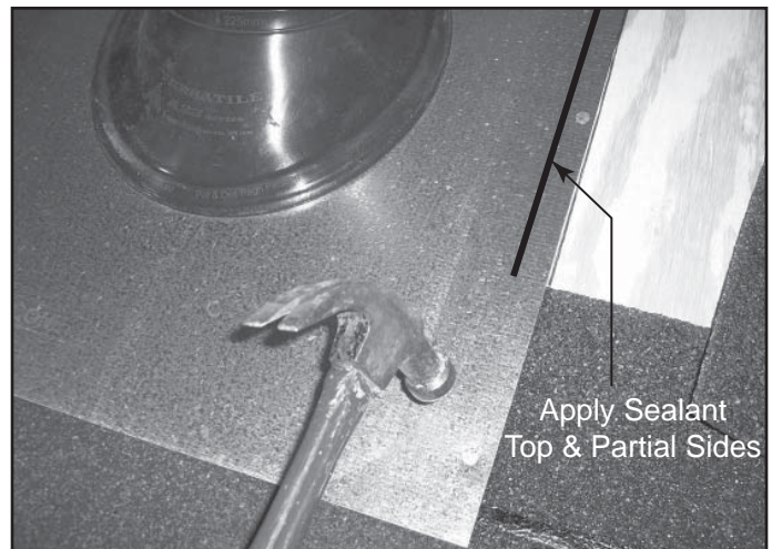
Figure 10.21 Slide Flashing Down, Secure & Apply Sealant
