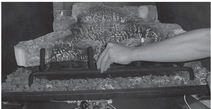
Figure 14.2 Placement of Vermiculite
