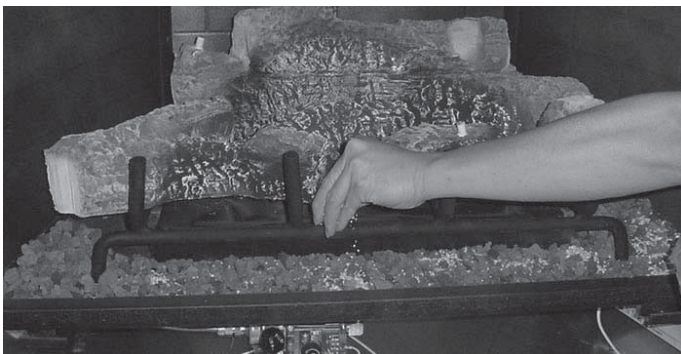
Figure 14.2 Placement of Vermiculite
