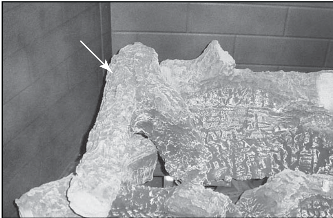
Figure 14.6 Placing Left Top Log
