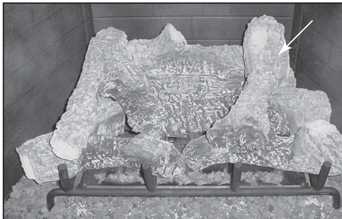
Figure 12.7 Placing Right Top Log
