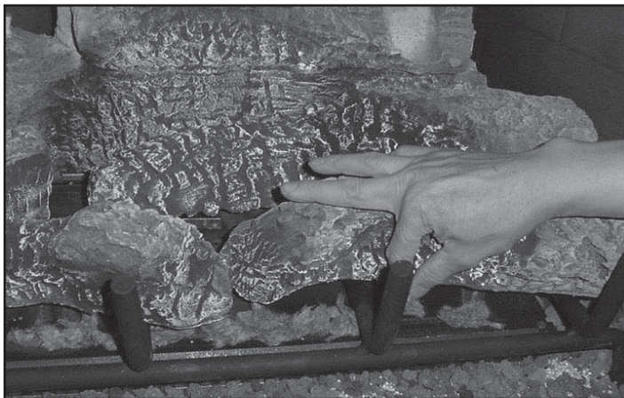
Figure 12.4 Placement of Rock Wool
