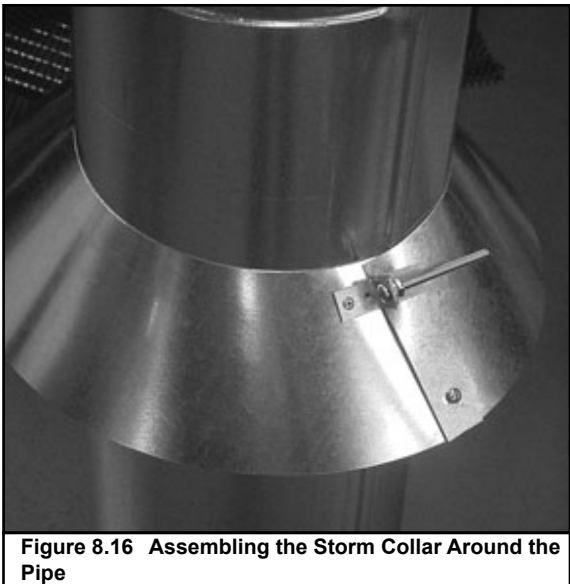
Figure 8.15 Assembling the Storm Collar
