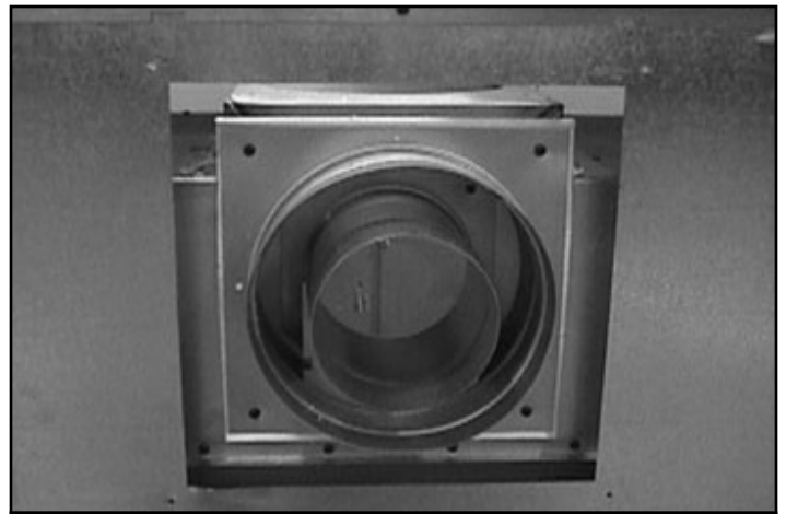
Figure 7.10 Place Outer Collar on Rear of Appliance
