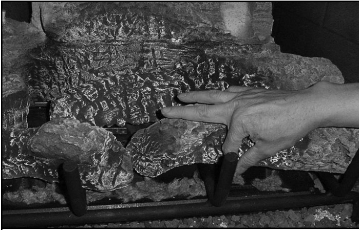
Figure 12.4 Placement of Rockwool
