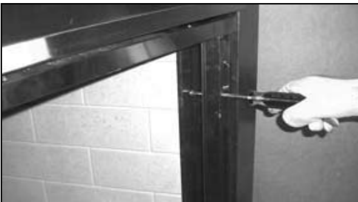
Figure 11.3 Loosen Refractory Retaining Strip
