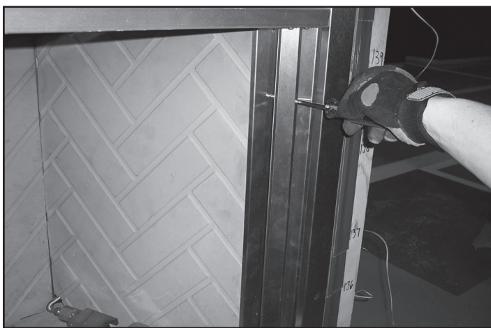
Figure 12.3 Loosen Refractory Retaining Strip
