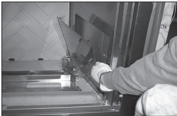
Figure 12.4 Remove Valve Access Panel
