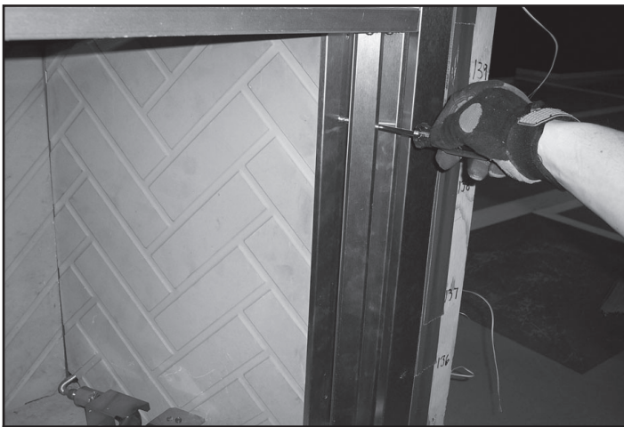
Figure 6.3 Loosen Refractory Retaining Strip
