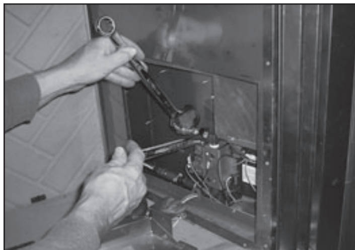
Figure 12.6 Turn off Gas Valve
