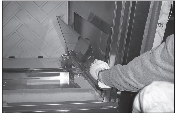
Figure 6.4 Remove Valve Access Panel
