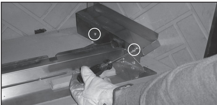
Figure 6.2 Remove Pilot Shield
