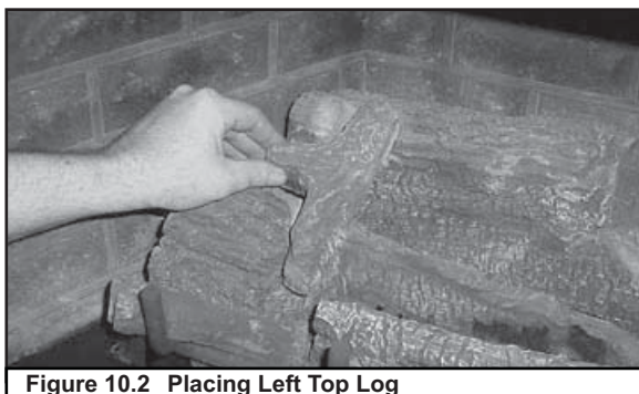
Figure 10.2 Placing Left Top Log
