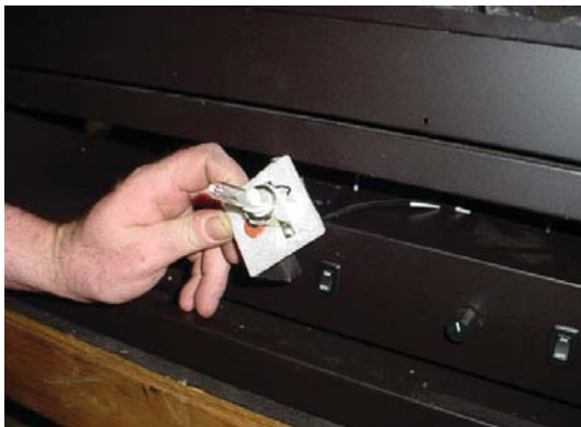
Figure 20 - Ember Bed Bulb Replacement
