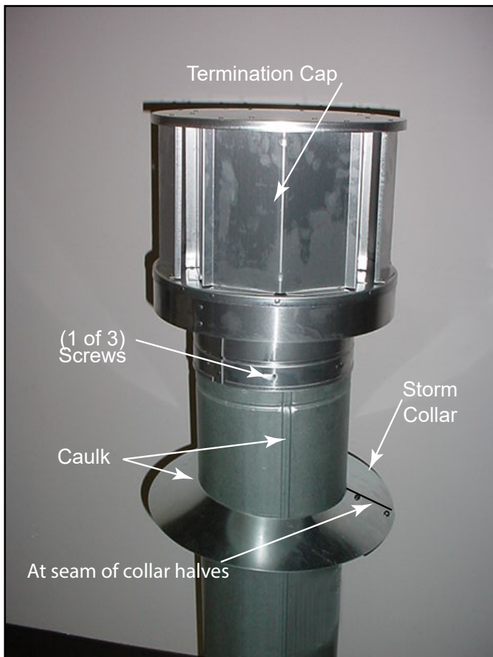
► Figure 20 Secure with Screws
