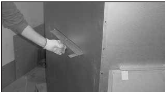
Figure 3.7 Bend Refractory Brackets Back Down
