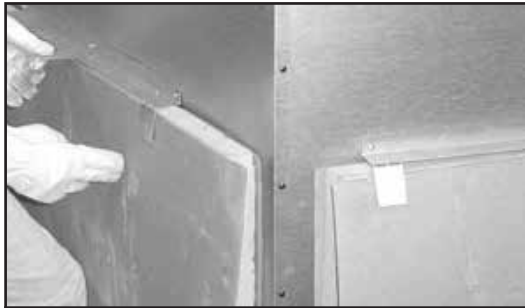
Figure 3.6 Unpack Back Refractory
