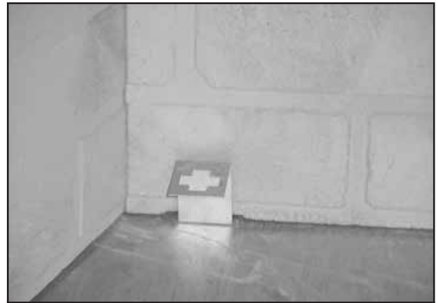
Figure 8.8 Grate Retaining Bracket in Place
