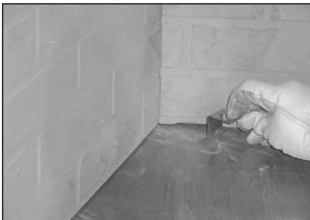
Figure 8.7 Slide Grate Retaining Bracket into Notch
