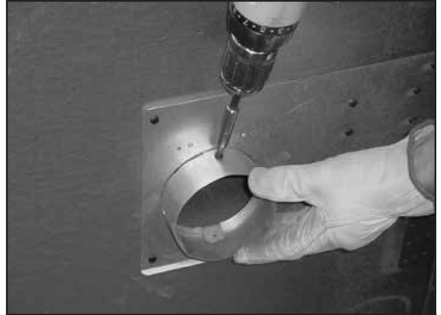
Figure 3.19 Attaching Outside Air Kit Collar
