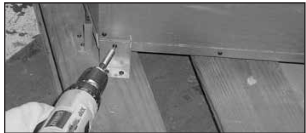
Figure 3.11 Removing Shipping Brackets
