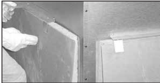
Figure 3.6 Unpacking Back Refractory
