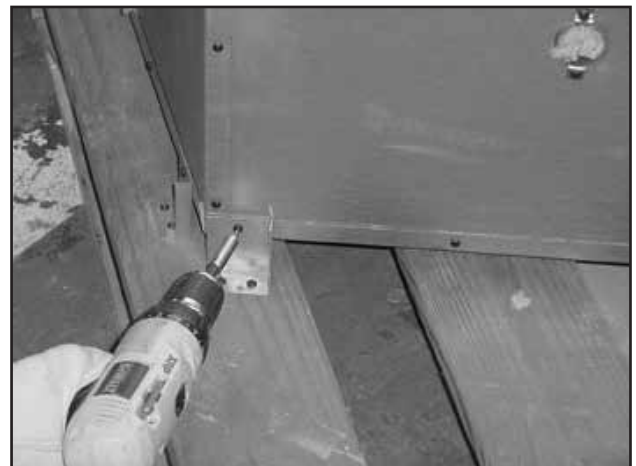
Figure 3.12 Removing Shipping Brackets
