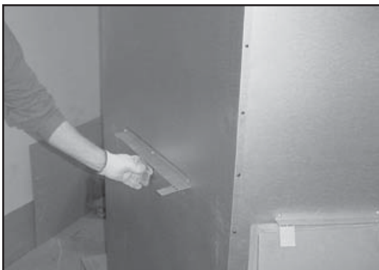
Figure 4.6 Bending Refractory Shipping Tabs Back Down
