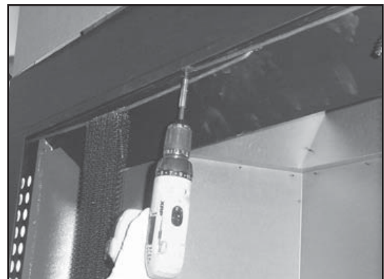
Figure 4.8 Removing the Screen Rods
