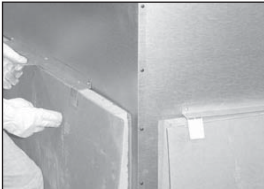
Figure 4.5 Unpacking Back Refractory
