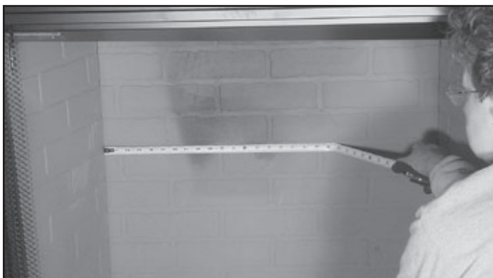
Figure 2.1 Measure Firebox
