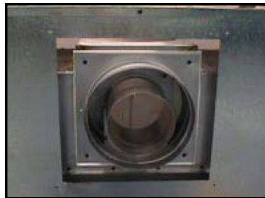
Figure 14 - Place Outer Collar on Rear of Appliance
