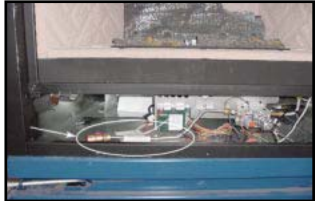
Figure 49 Flex Connector & Manual Shutoff Valve
