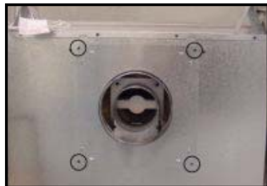
Figure 15 - Place Plate on Rear of Appliance
