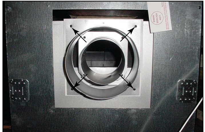
Figure 7.8 Attach Outer Collar
