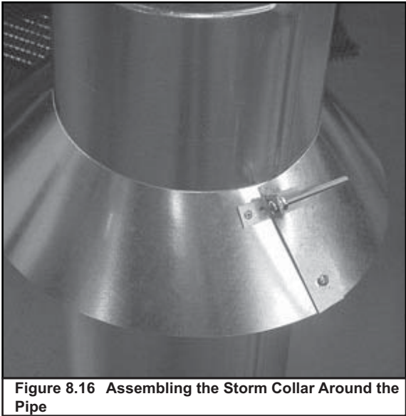
Figure 8.15 Assembling the Storm Collar
