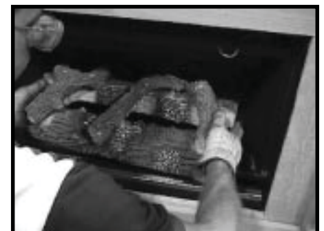
Figure 35 - Log Removal
