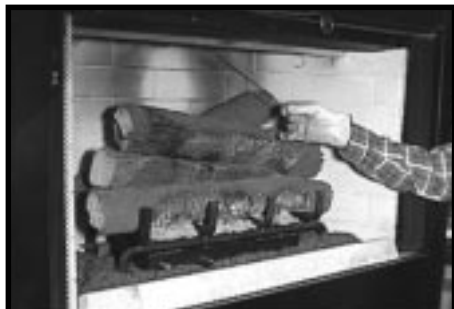
Figure 12 - Checking for Spillage
