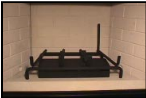
Figure 5 - Placing the Grate Assembly
