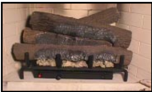
Figure 10 - Placing Mineral Wool
