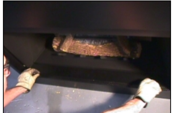
Figure 27 - Access Panel Removal
