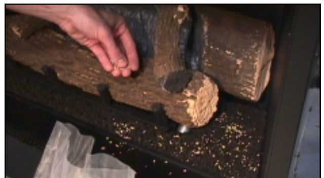
Figure 22 - Placing the Vermiculite
