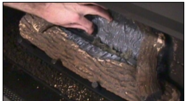
Figure 23 - Placing the Rock Wool
