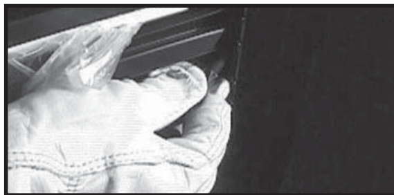
Figure 18 - Upper Grille Panel Removal
