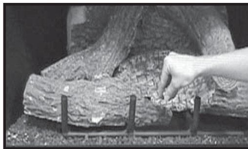
Figure 23 - Placing the Vermiculite
