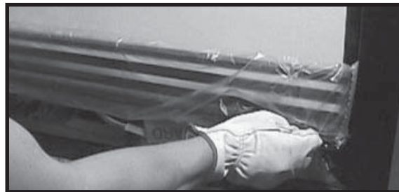
Figure 19 - Control Access Panel Removal
