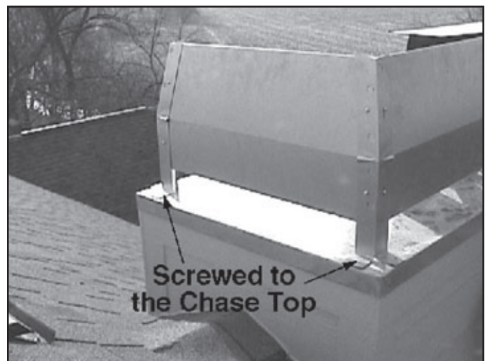
Figure 19 Shroud Attached to Top of Chase
