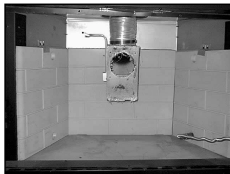
Figure 6 - Draft Hood Attachment
