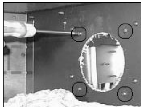
Figure 5 - Draft Hood Removal
