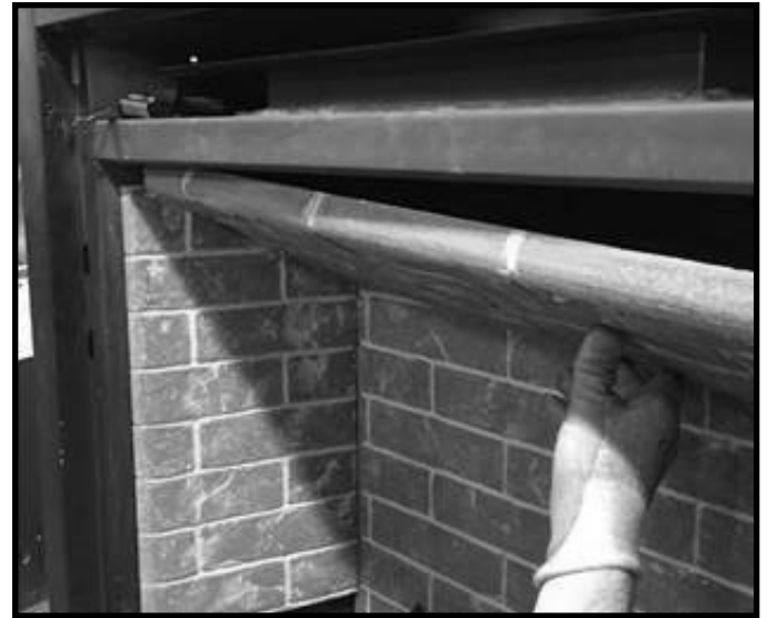
Figure 11.4 Install Top Refractory Panel
