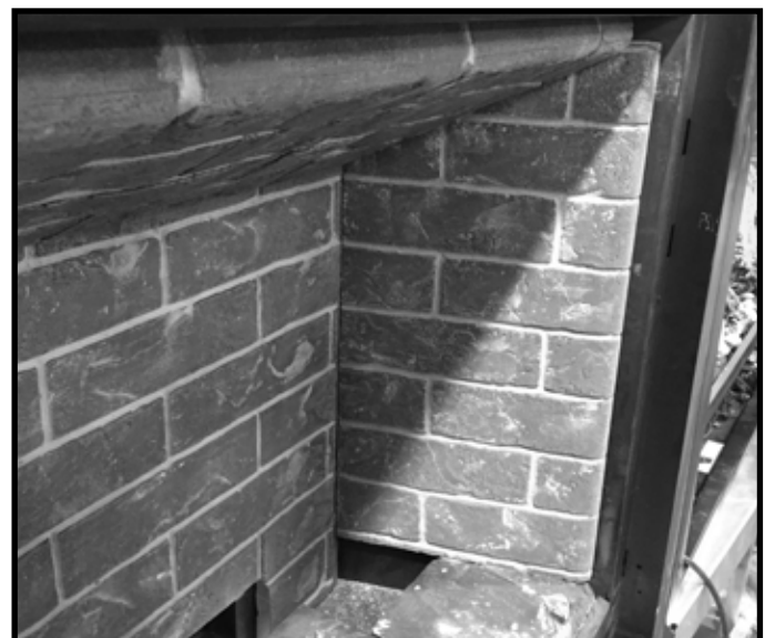
Figure 11.6 Right Refractory Panel Installed
