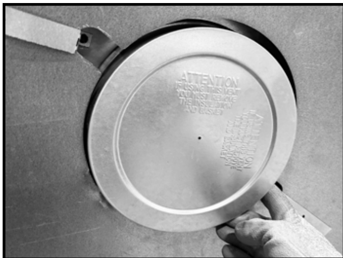
Figure 6.10 Fold the straps away from cap. Remove seal cap utilizing cutouts.
