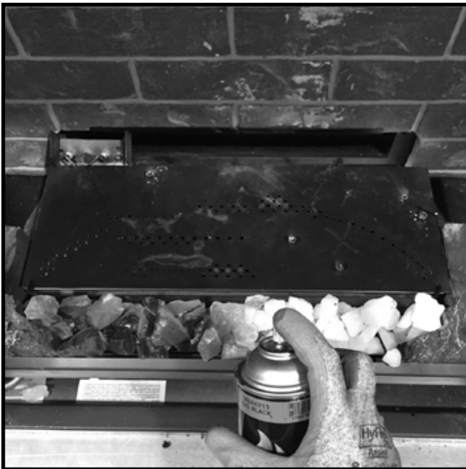
Figure 11.18 Paint Teco-Sil
