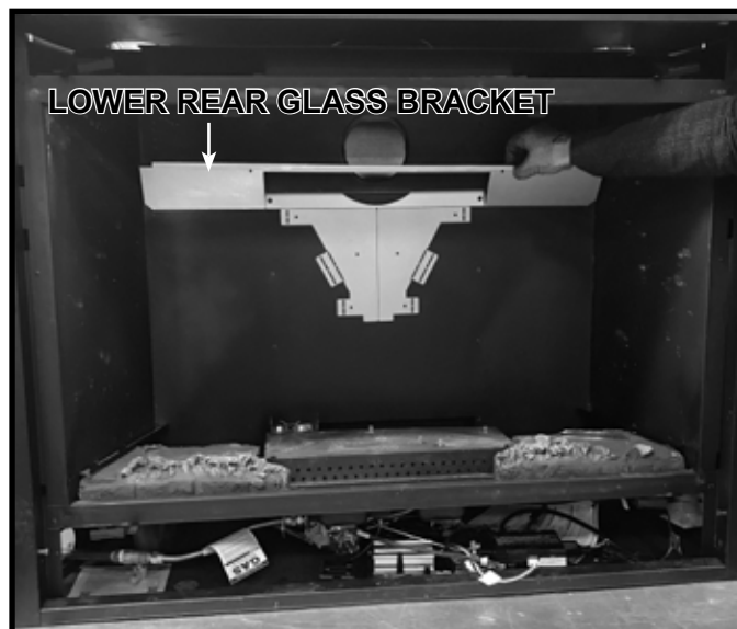
Figure 11.8 Removing Lower Rear Glass Bracket
