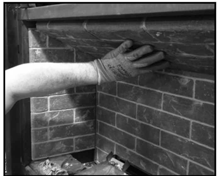
Figure 11.5 Install Right Refractory Panel
