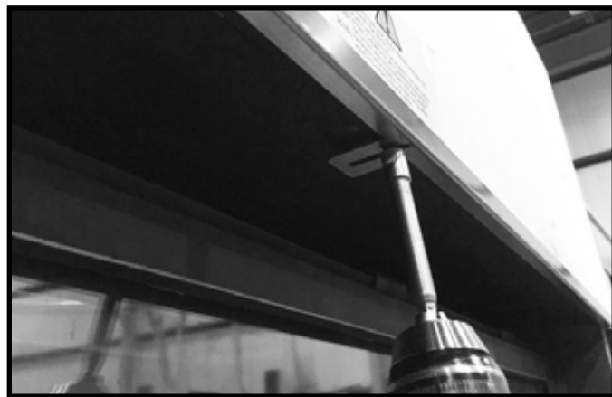
Figure 10.5 Install Trim Ring
