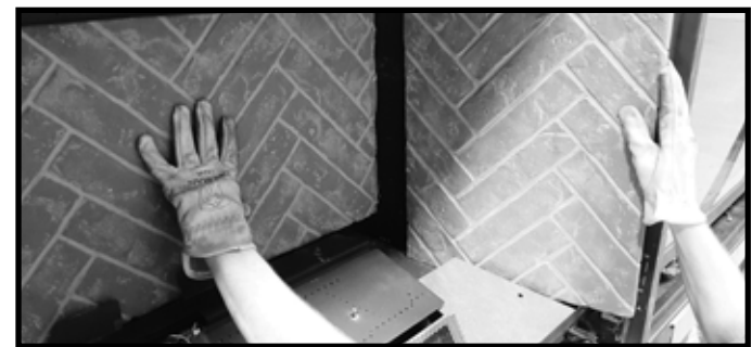
Figure 11.3 Install Side Refractory Panel (Right Side Shown)
