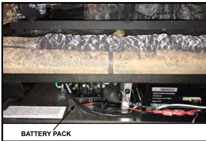
Figure 3.8 Battery Pack Installed
