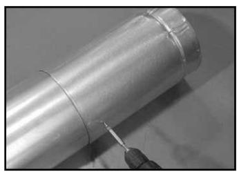
Figure 7.7 Screws into Slip Section
