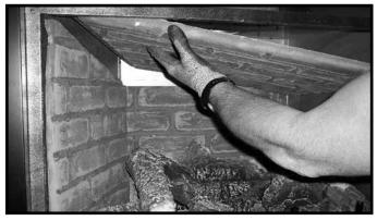
Figure 4.15 Remove Top Refractory
