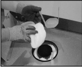
Figure 6.4 (Generic Fireplace Shown) Remove the insulation basket and white insulation from the center vent
