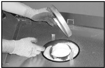
Figure 6.3 (Generic Fireplace Shown) Remove the seal cap.
