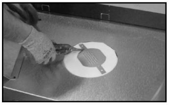
Figure 6.1 (Generic Fireplace Shown) Cut the seal cap strap across the rectangles next to the disk.
