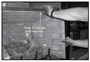
Figure 4.14 Remove One Side Refractory
