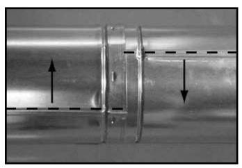
Figure 7.10 Rotate Seams for Disassembly
