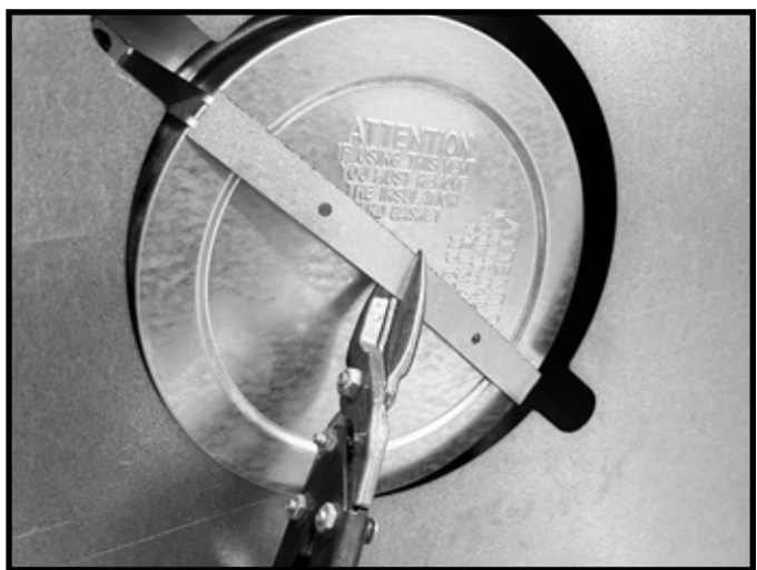
Figure 6.13 Cut the metal retaining band.
