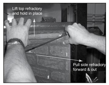
Figure 4.17 Remove Side Refractory
