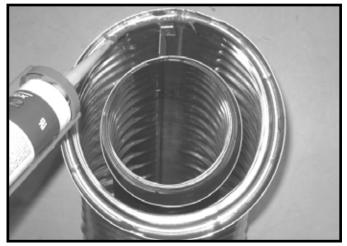
Figure 7.1 High Temperature Silicone Sealant
