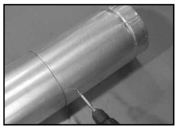
Figure 7.7 Screws into Slip Section
