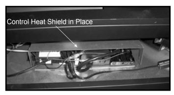
Figure 11.4 Control Heat Shield - Installed
