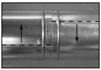
Figure 7.10 Rotate Seams for Disassembly
