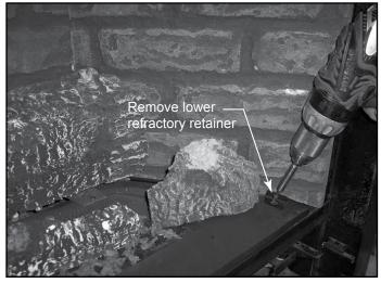
Figure 4.17 Remove Refractory Retainer
