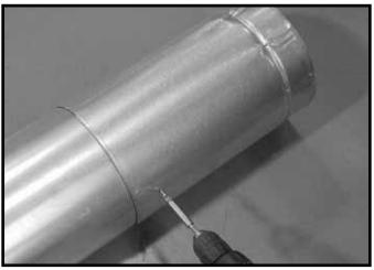
Figure 10.7 Screws into Slip Section
