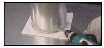
**Figure 9.6** To attach the first section of vent pipe, make sure to use the fiberglass gasket in the manual bag to seal between the first vent component and the outer fireplace wrap. Use 2 self tapping screws to secure the gasket to the outer wrap.
