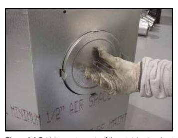
**Figure 9.9** Fold the center parts of the retaining band out and use to remove the seal cap.
