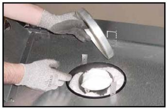
Figure 9.3 Remove the seal cap.
