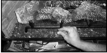
Figure 14.4 Placement of Vermiculite
