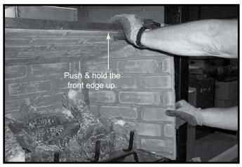
Figure 7.9 Remove One Side Refractory
