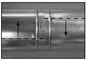
Figure 10.10 Rotate Seams for Disassembly
