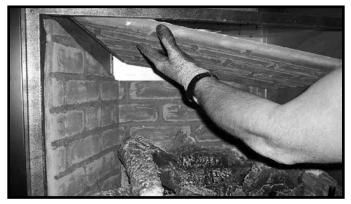
Figure 7.10 Remove Top Refractory
