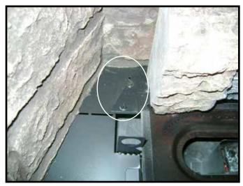
Figure 3.7 Remove Screws from Log Tabs
