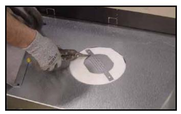
**Figure 9.1** Cut the seal cap strap across the rectangles next to the disk. For rear vent, skip this step.
