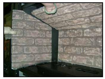
Figure 3.2 Top Refractory Removal
