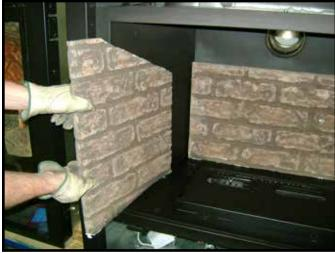
Figure 3.3 Side Refractory Removal
