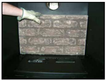
Figure 3.4 Back Refractory Removal
