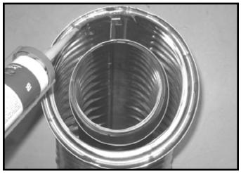
Figure 10.1 High Temperature Silicone Sealant
