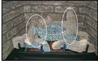
Figure 3.5 Remove Top Two Logs
