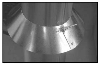
Figure 10.13 Assembling the Storm Collar Around the Pipe
