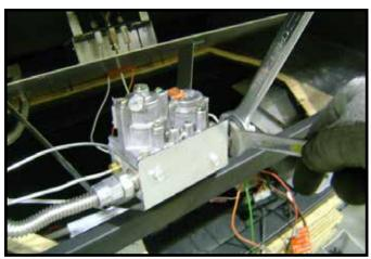
Figure 11.4. Disconnect Gas Valve
