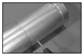
Figure 10.4 Screws into Slip Section
