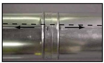
Figure 10.8 Align and Disassemble Vent Sections
