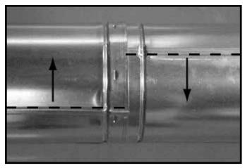
Figure 10.7 Rotate Seams for Disassembly
