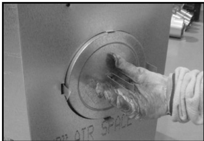
Figure 6.10 Fold the center parts of the retaining band toward the center as shown. Remove the seal cap.
