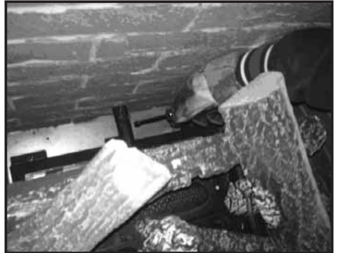
Figure 1. Air Shutter Location
